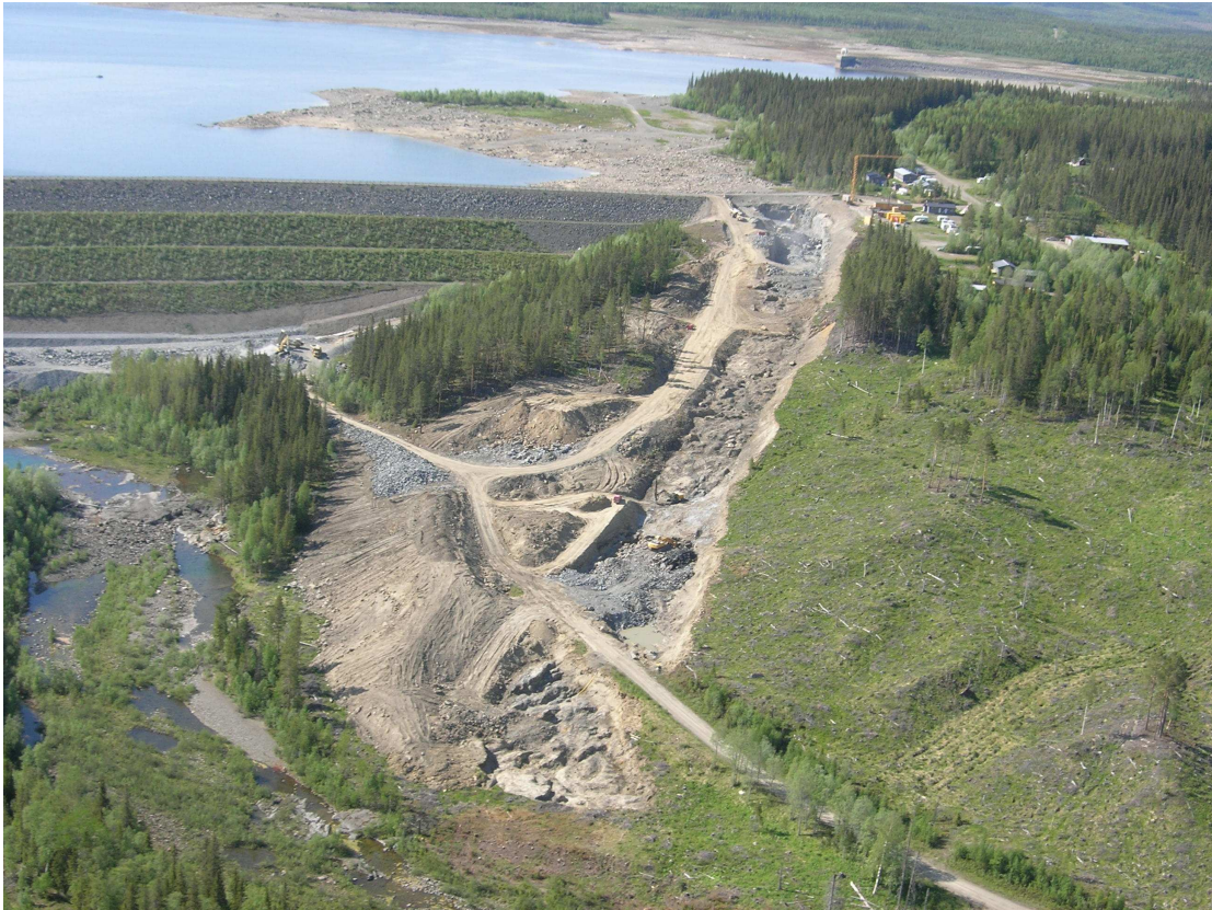
Figure 8. On-going reconstruction to provide the Håckren dam with a new spillway to upgrade the discharge safety. (Photo: Vattenregleringsföretagen, 2006)
