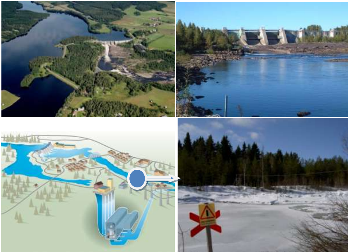
Pictures showing the area the Sornorrfors dam and the dam and spillway from downstream.
